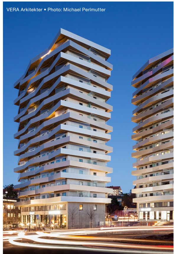
Flats in Stockholm, Sweden
